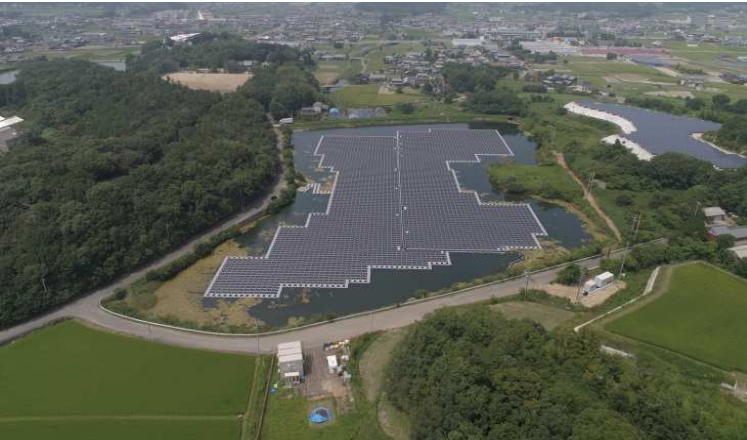
Kagawa Mitakabeike solar power plant 1.5MW
