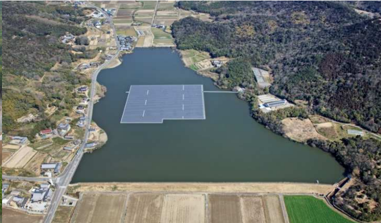
Kagawa Nomaike solar power plant 2.4MW
