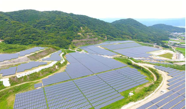
Shizuoka Izunokuni-shi Kitaema solar power plant 11.3MW
