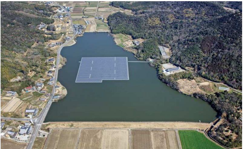
Kagawa, Sanuki Nomaike solar power plant
